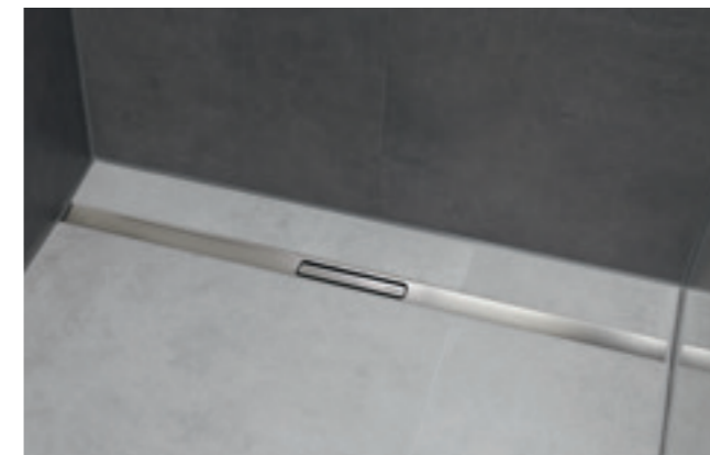
↑ A simple tap of the finger is all it takes to remove the floating waste plug above the integrated comb insert.
